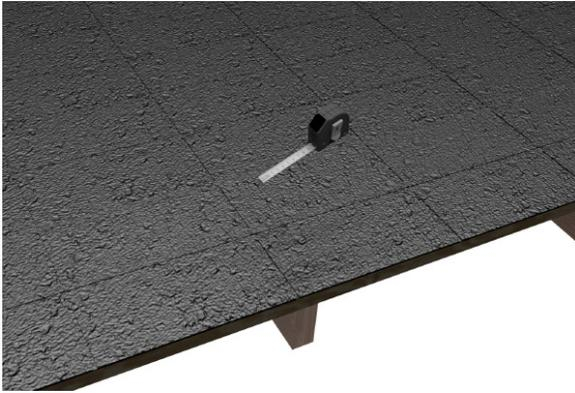
Locate the rafters and snap horizontal and vertical lines to mark the installation position for each EverFlash flashing. Drill a pilot hole (1/4" diameter) for the lag bolt. Backfill with appropriate sealant. Always consult a professional roofer to ensure integrity is maintained.
