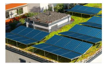
K2 GreenRoof Vento ensures stability and - thanks to the greater distance from module to roof - reliably prevents the modules from being shaded by excessive vegetation.
