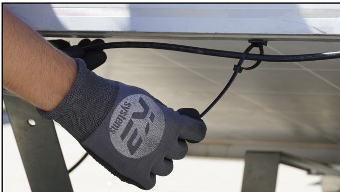
Hellermann Tyton Edge Clip and Cable Ties example of installation
