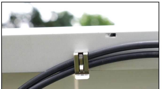
Wiley cable clips example of installation
