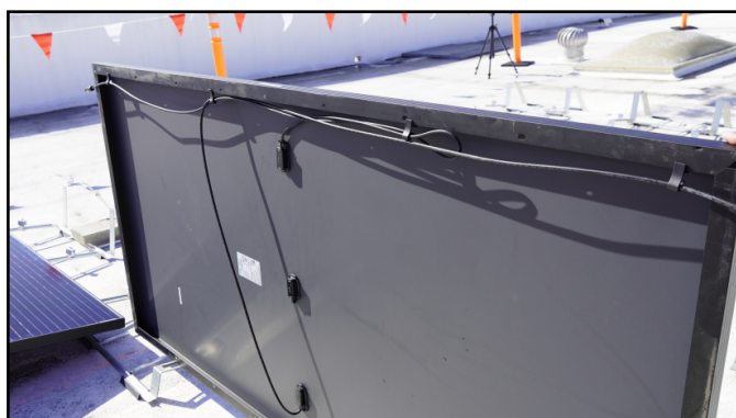
K2 Dragon Clip example of installation
