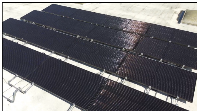
All wiring managed under module; required conduit, raceways, and cable ties are not shown in the example above.
