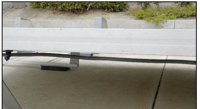
Hellermann Tyton Edge Clip and Cable Ties example of installation
